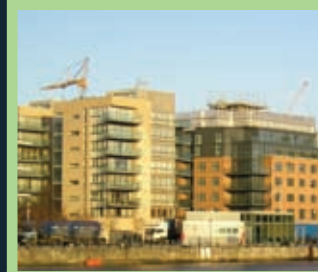
North Wall Quay / 180
